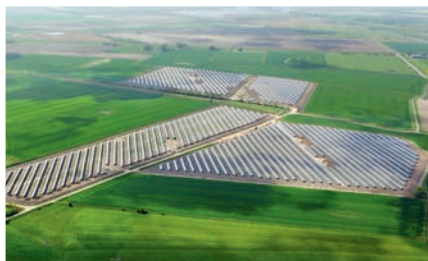
Solarpark Meldorf, 7.655 kWp
